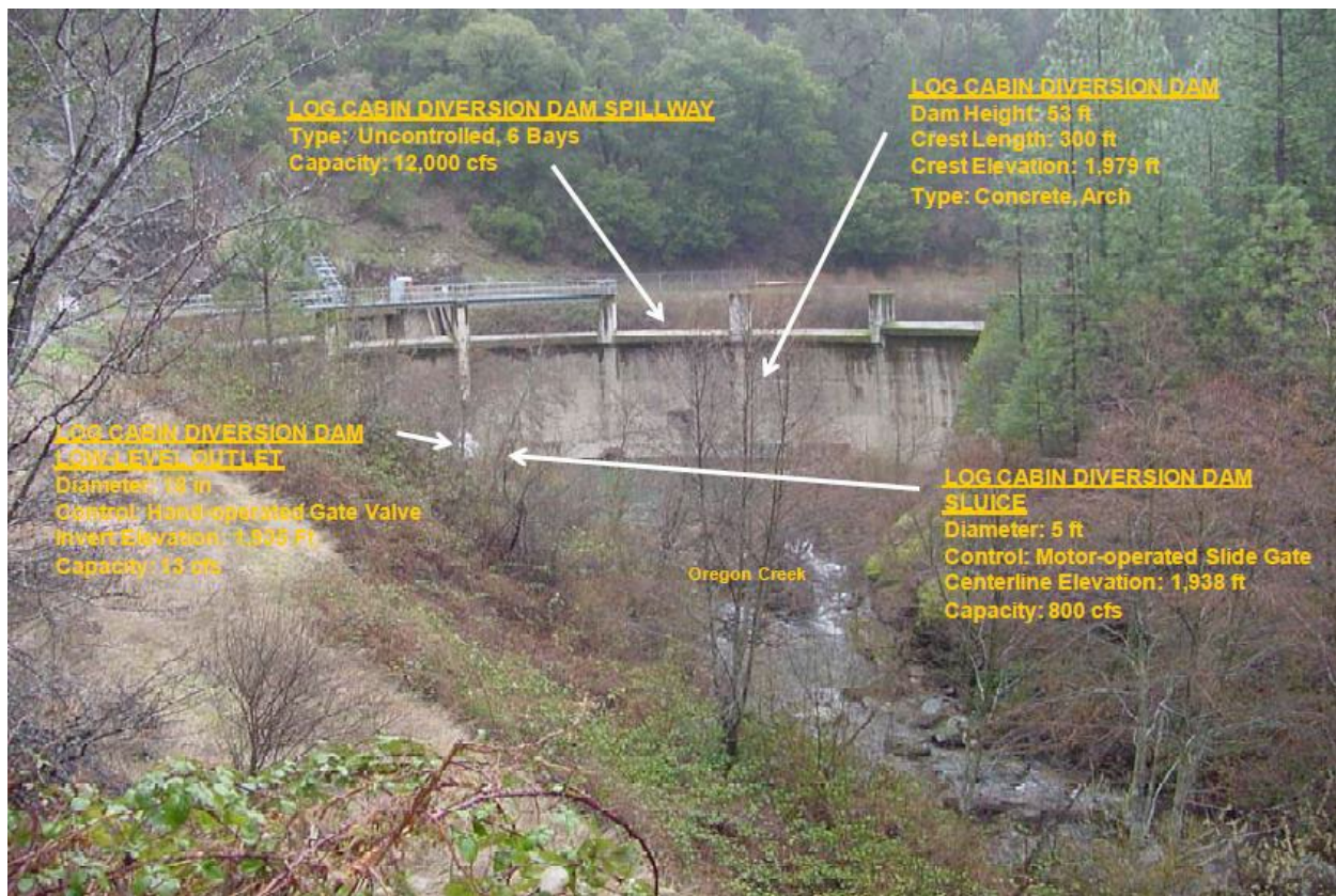
Figure 3. Log Cabin Diversion Dam on Oregon Creek. Source: YCWA (2010).
